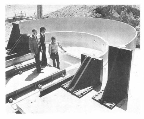
DAVE BICKEL (9335), RICH-ARD YOSHIMURA (5433) AND BOB LUCAS (9335) inspect target structure for turbine fragment test—a full-sized model representing a portion of the low pressure section of a large steam turbine. Inner steel ring was heated to about 100°F to approximate actual turbine operating conditions.
